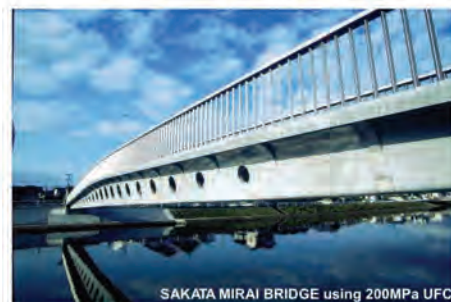
SAKATA MIRAI BRIDGE using 200MPa UFC
