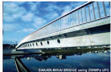
SAKATA MIRAI BRIDGE using 200MPa UFC
